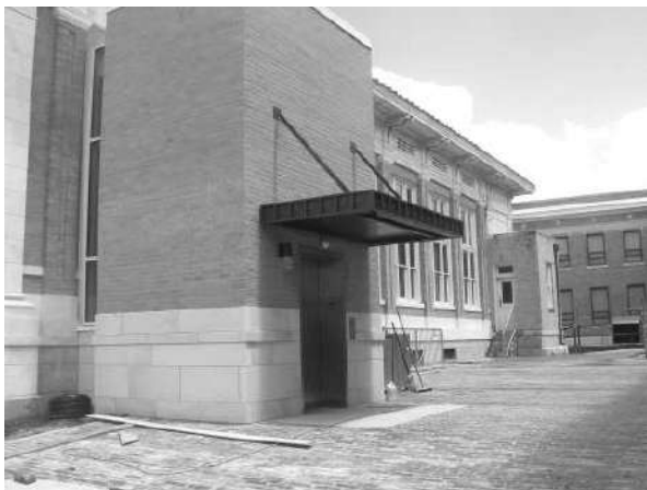
New elevator on the side of the building
