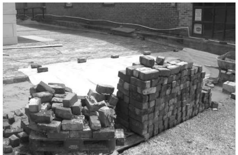
Original brick pavers waiting to be reinstalled
