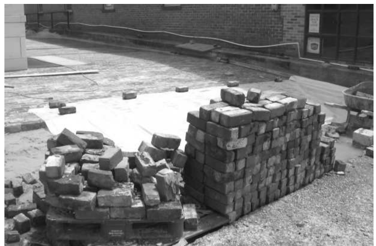
Original brick pavers waiting to be reinstalled
