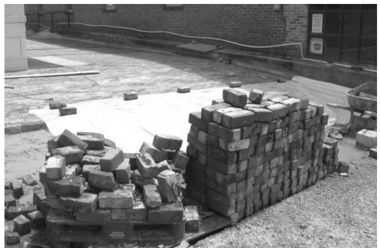
Original brick pavers waiting to be reinstalled
